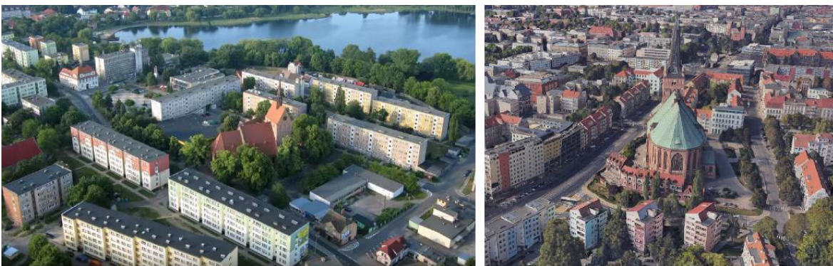
Fig. 4. Historical old-town areas of Nowogard (to the left) and Szczecin (to the right), featuring multi-family housing blocks. Source: Google maps
