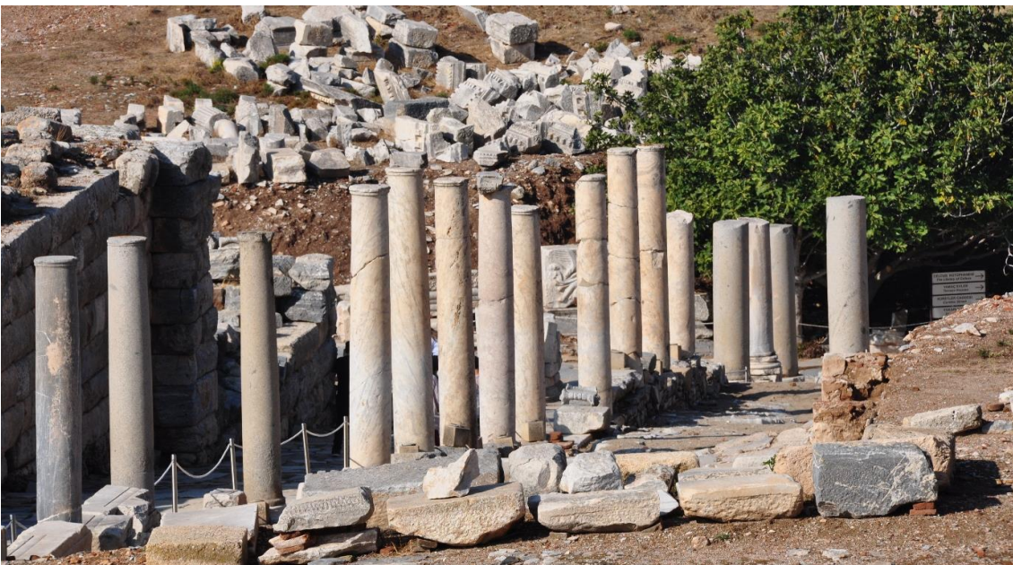
Fig. 17. Anastylosis of a street colonnade in Ephesus (Turkey). Source: author's photo
