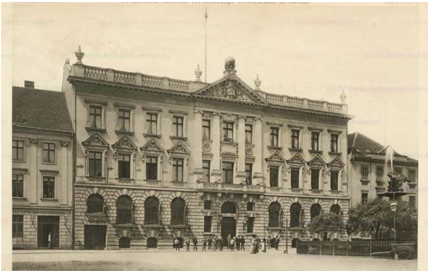
Fig. 6. The view of the Palace façade, the state from 1894. Source: [5, p. 54]
