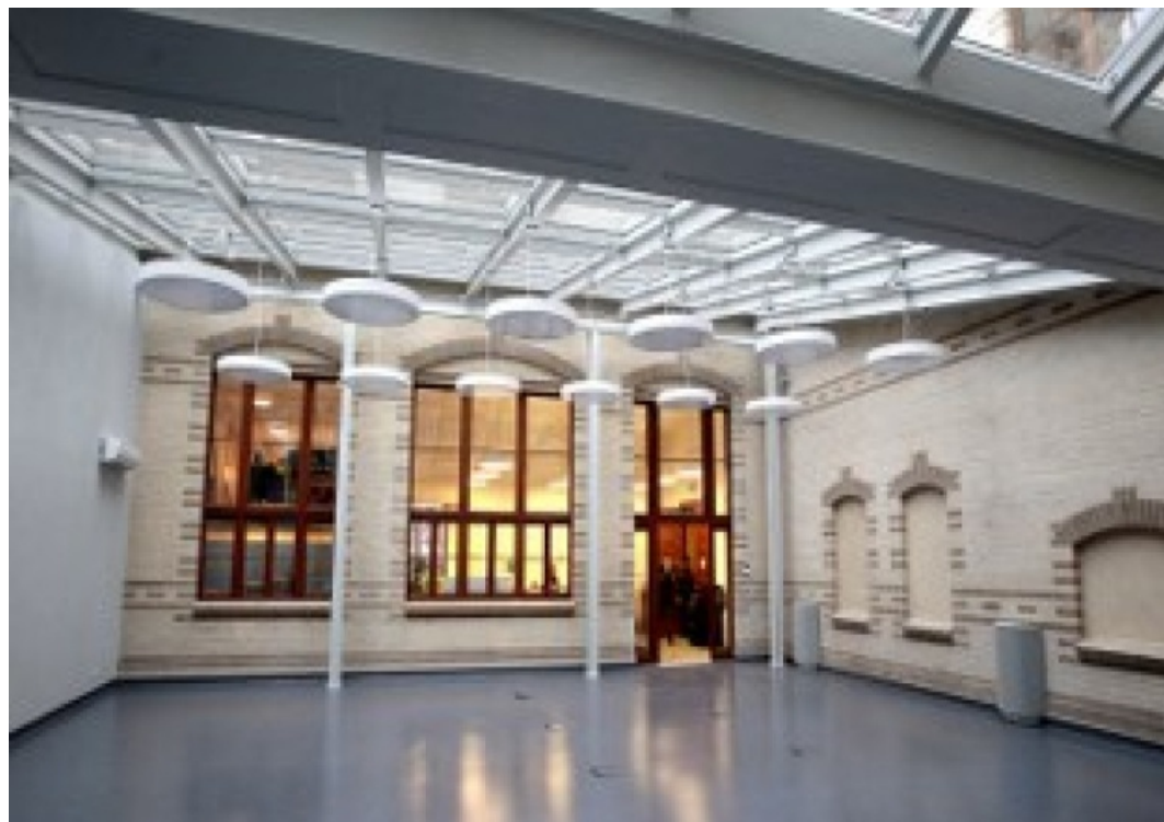
Fig. 12. The sheltered part of the north courtyard included into the existing premises of the multimedia library on the 1st floor level. Source: photog. by M. Tuszyński
