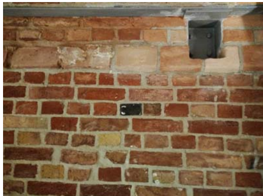
Fig. 14. Using mortar painted into color of wall instead of bricks in unusual size. Source: K. Wierzbicki, October 2016
