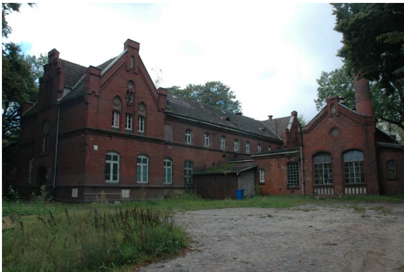
Fig. 6. Old Military Laundry before rebuild. Source: J. Stawicka, September 2011
