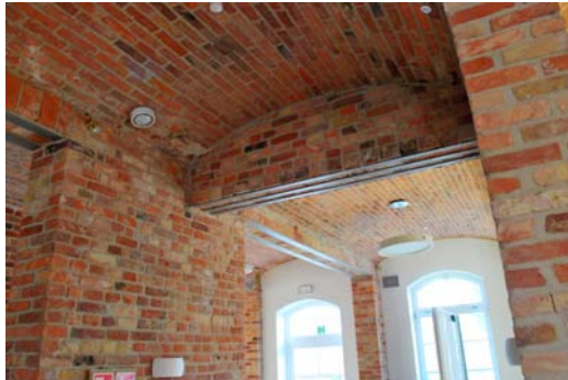
Fig. 11. Downstand beam instead of a load-bearing wall. Source: R. Cypryański, February 2017
