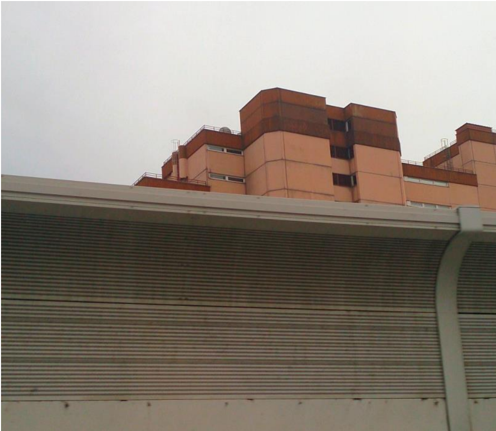
Fig. 2. An acoustical barrier with a residential building behind it. The building features a minimal number of windows on the side bordering a noisy road – Vienna, Austria. Source: author's own photo
