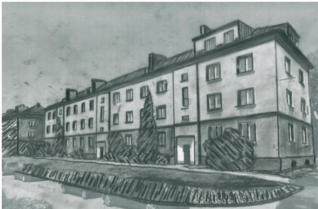
Fig. 9. Block of flats on Radości st. Dormers do not harmonize with building. Source of figure: Author.
