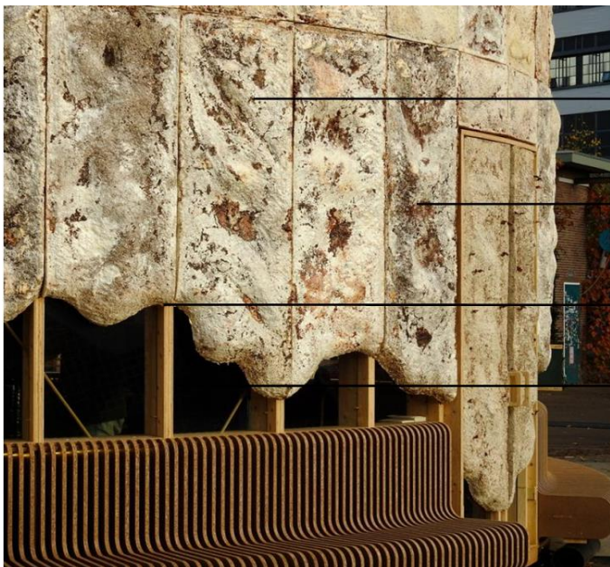
Fig. 4. Close-up of a detail of the wooden construction and panels made with MBC of The Growing Pavilion. Source: photo Eric Melander
