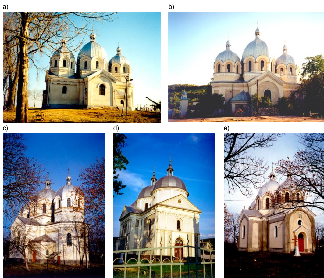
Fig.10. Three-domed stone churches built in 1772-1918 in the territory of Galicia: a) Mykolayiv, Patronage of the B. V. Mary Church, 1903; b) Grybovychi, Sts. Kosmas and Damian Church, 1897; c) Perehnoyiv, Presentation of the B. V. Mary Church, 1907; d) Chervone, Sts. Kosmas and Damian Church, 1886; e) Utishkiv, Synaxis of the B. V. Mary Church, 1908. Source: Author.
