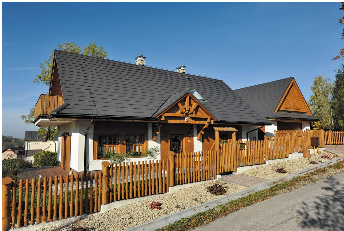
Fig.2 House by Studio Atrium, named Koliba, source: photo Justyna Juroszek
