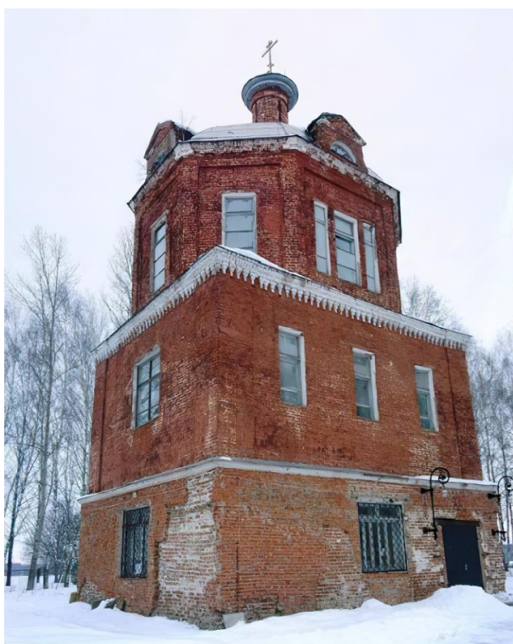
Fig. 2. Ruins of the Church before the start of reconstruction. Source: website of the Church of the Life-Giving Trinity in the village Goretovo.
