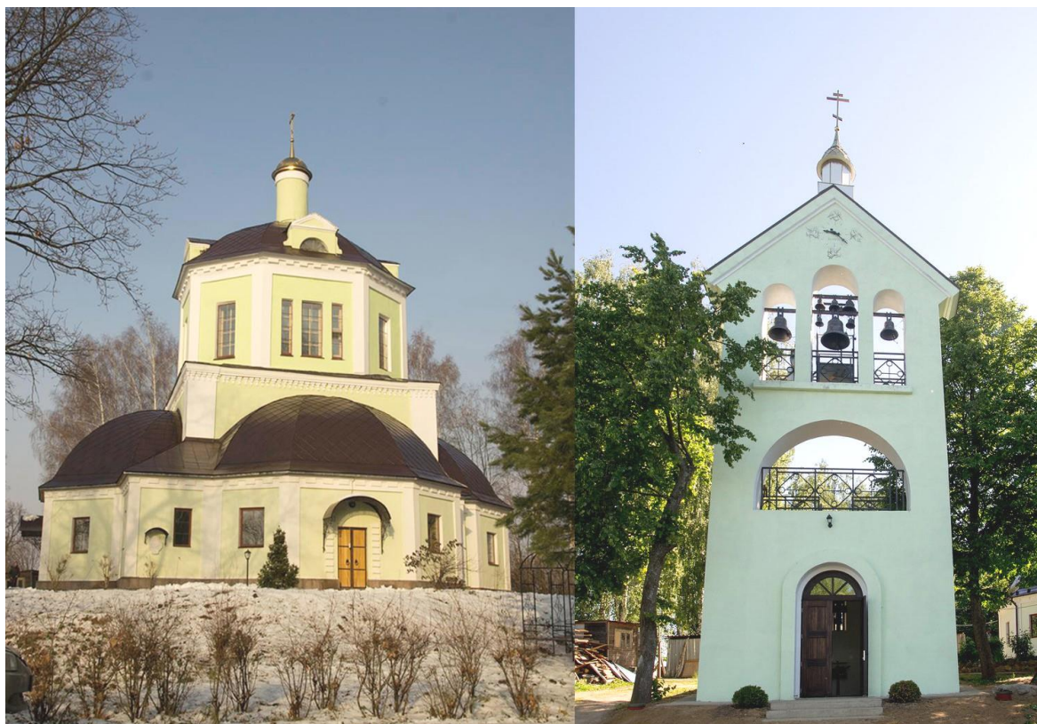
Fig. 4. Restored church. Belfry-'milovid'. Source: website of 'Kapitel' magazine
