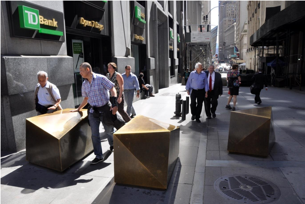
Fig. 11. Road barrier at the entry to Wall Street made of bronze NoGo elements, 2013.
