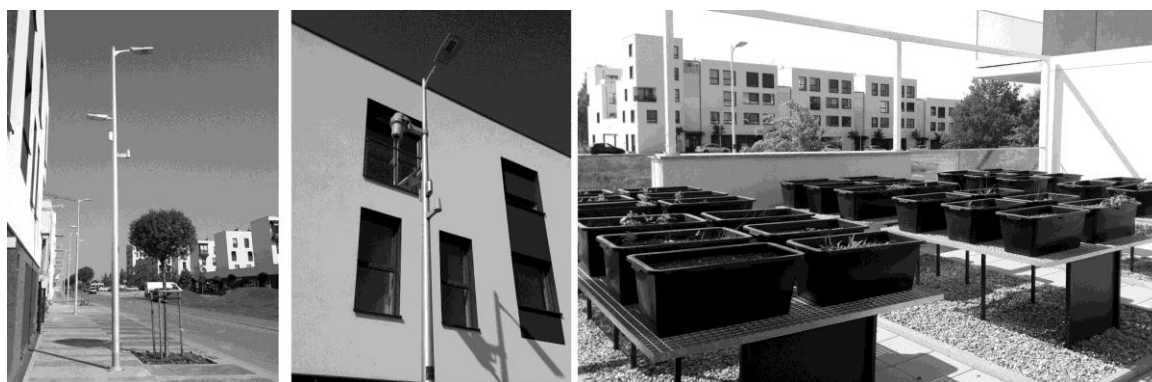
Fig. 1. Right and middle - street lighting - in the frontage of Krystyna and Marian Barski Street. Visible effects of the integrated design of technical, road and green infrastructure. Photos: Paweł Horn. Source: (Horn, P. 2019. P. 125). Left – gardening pots for dwellers of one of the estate's multifamily quarter. Photo: ibidem, p.174
