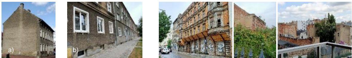
Fig. 2. Architecture that has not been renovated after the Second World War. (a) Nowe Warpno, (b) Gorzów Wielkopolski, (c) Łódź
