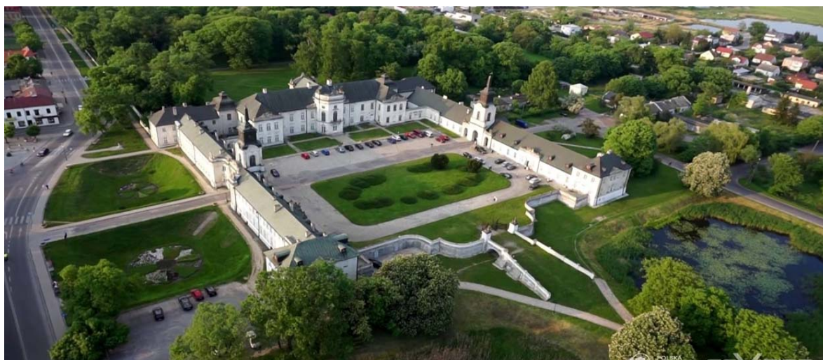
Fig. 15. View of the Potocki Palace in Radzyń Podlaski with its surroundings and water resources. Source: Material of Lublin University of Technology (archive).
