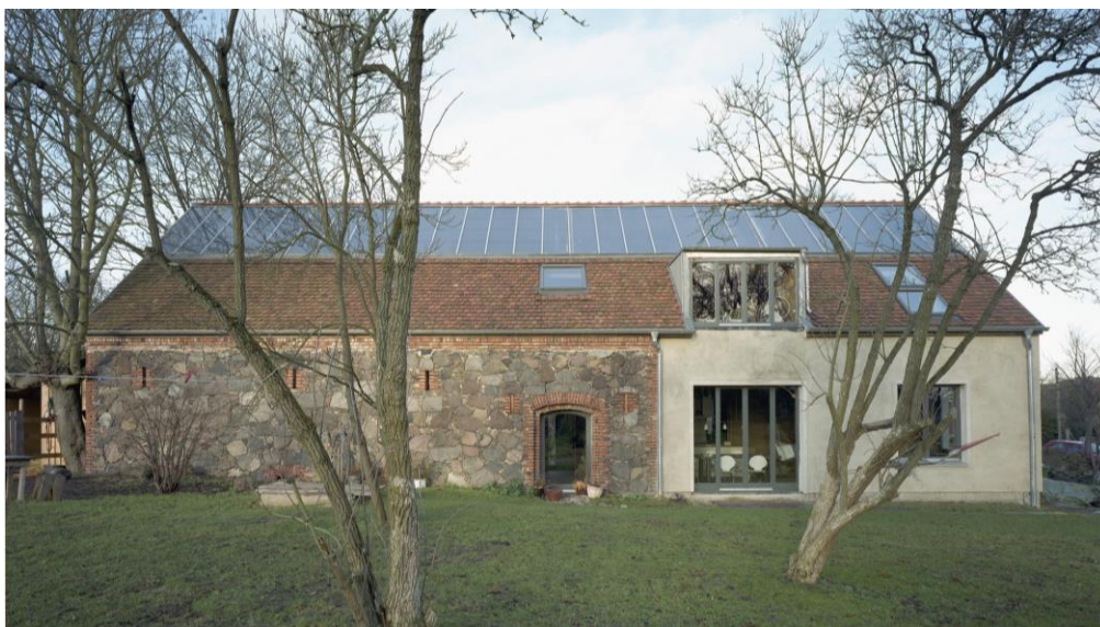
Fig. 5. An example of the successful adaptation of a farm building in Germany for the housing function. The project by Roswag Architekten. Source: [17]
