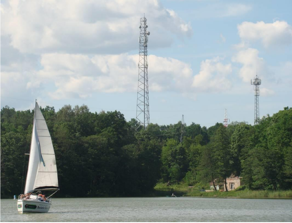
Fig. 3. Mobile telephone masts on Nidzkie Lake. Source: W. Gadomska
