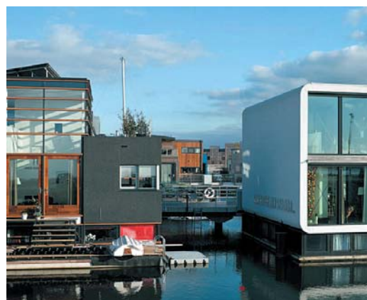
Fig. 4. A different nature of the two community housing parts. Waterbuurt East. Source: [1]
