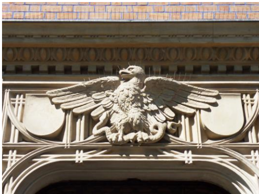
Fig. 7. Stone eagle fighting with the snake placed on portico input pharmacy in the House in the Main Market No. 45 in Krakow. Source: A. Jurek
